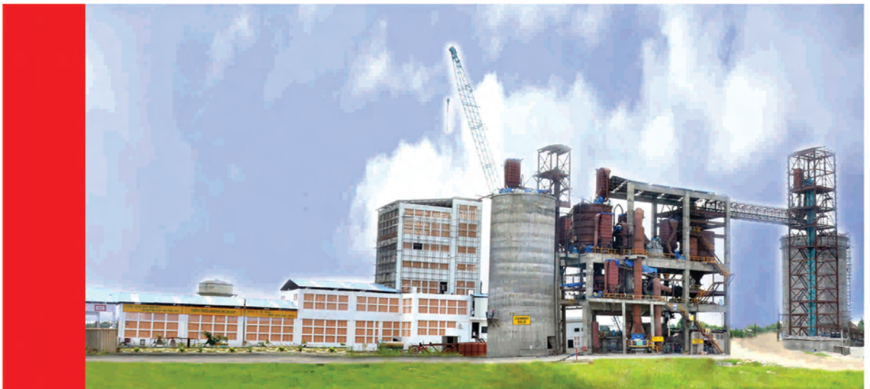
New Grinding Unit under construction in Aligarh (UP).
